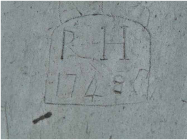
Figure 18 Plumber's mark from 1748. Many historic roofs have unique or distinctive markings.
