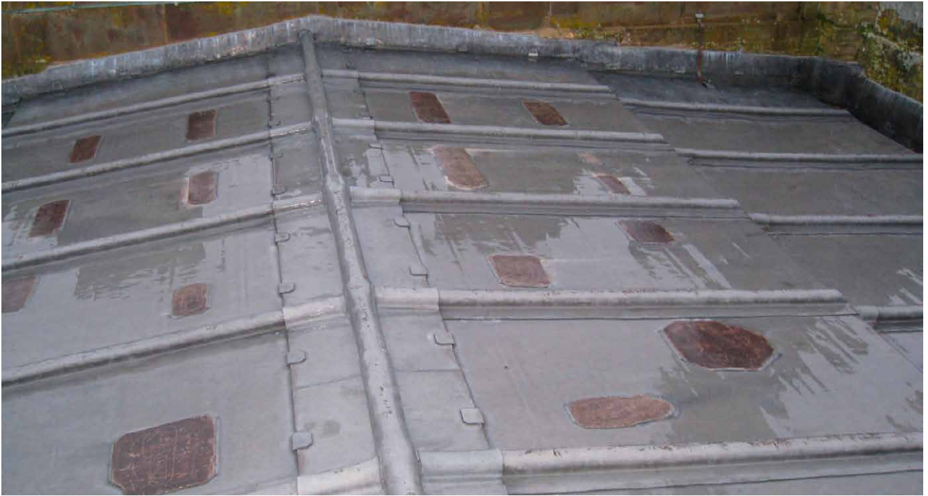
Figure 8 Repaired lead sheeting incorporating graffiti from before the First World War.
