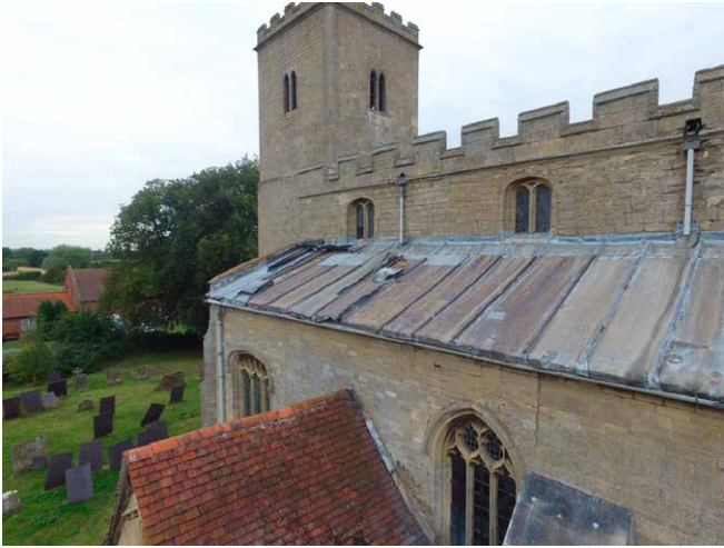
Figure 4 Thieves partially stripped this church of lead, leaving a lot of damage.
