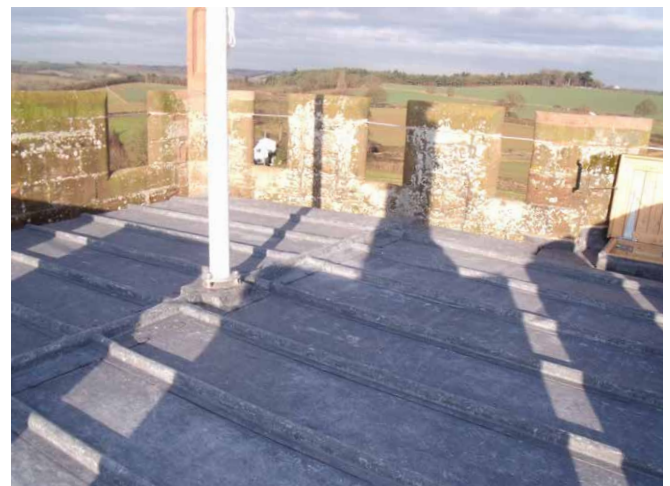
Figure 3 1960s lead roofing patched to recommended Lead Sheet Association standards.
