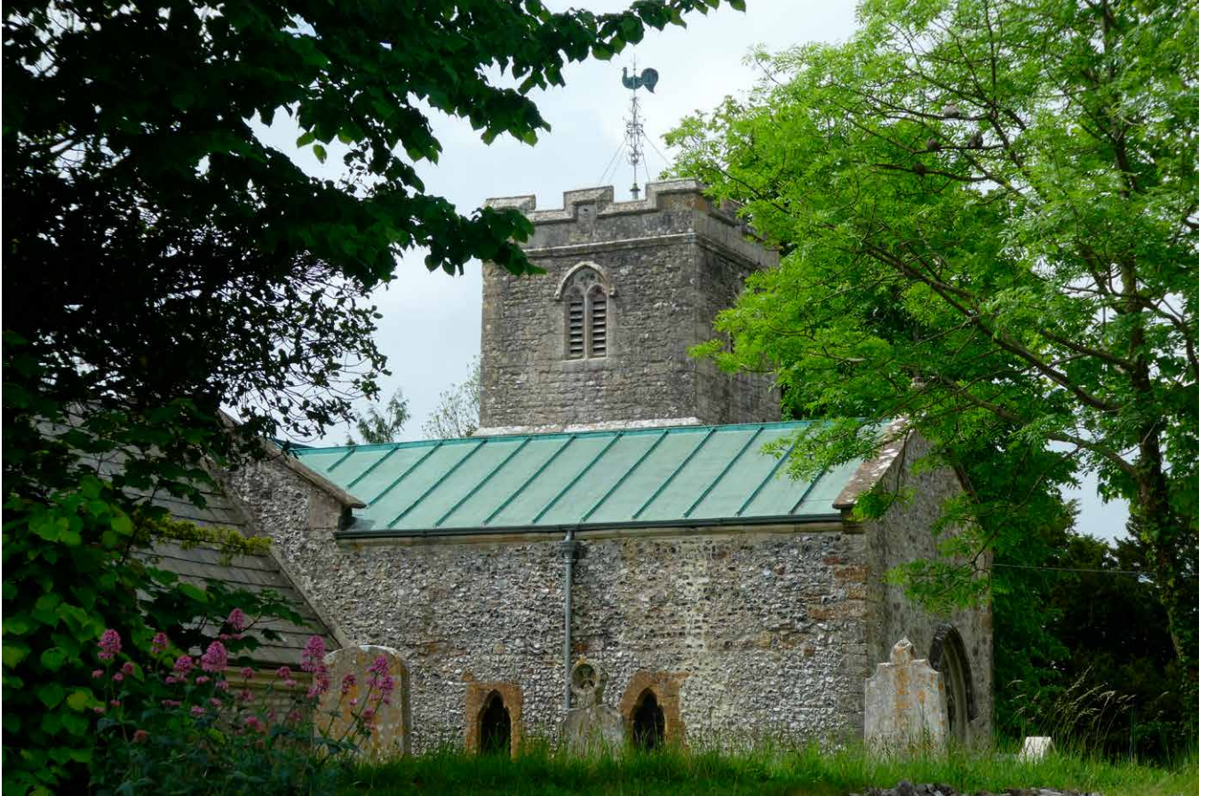
Figure 12 A rural church with a copper roof of distinctive green colour.
