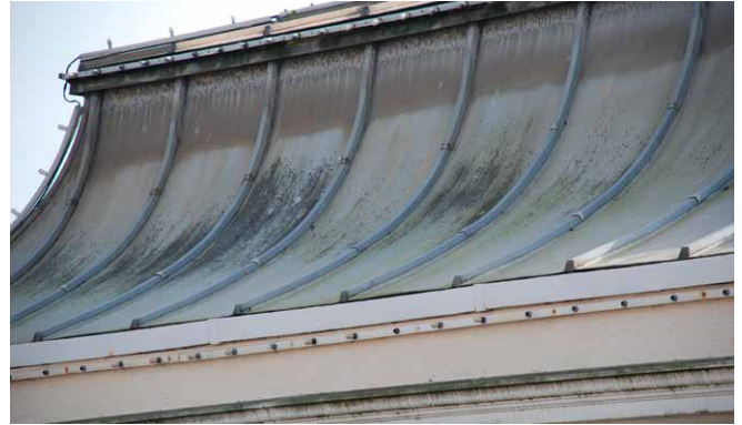
Figure 14 A zinc roof which has weathered over time.
