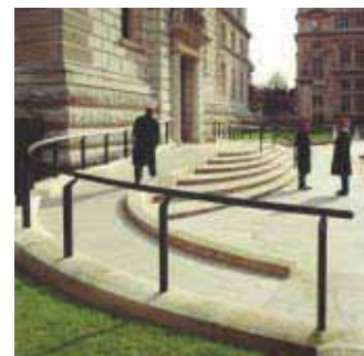
The refurbishment of the Government Offices, Great George Street, in Westminster has included disabled access at both entrances. High-quality design complements the refurbishment of the historic elements.
