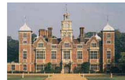
A lift at Blickling Hall has been located within one of the turrets without damage to the internal structure.
