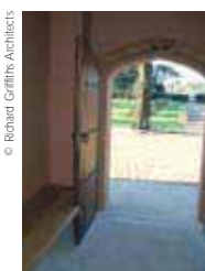
At Eastbury Manor the entrance lobby area can be raised as a ramp to overcome the existing level change while allowing the entrance doors to open inwards when the ramp is not in use.
