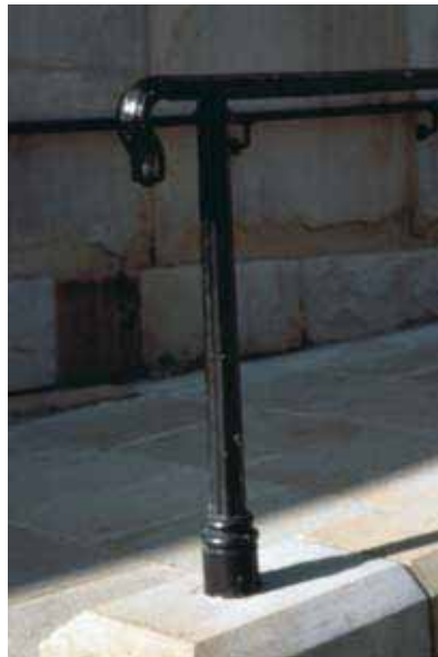
The new handrail at Huddersfield station is in keeping with its context.
