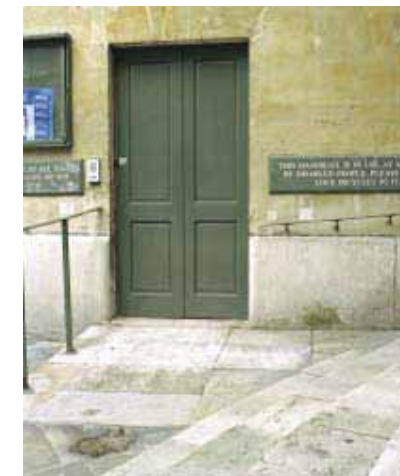
All Souls Church, Langham Place, London. An inconspicuous handrail leads up the side of the porch steps and a shallow ramp to a side entrance leads to a lobby and passenger lift that serves the church above and the refectory and hall in the crypt. Visual impact upon the porch, which is of critical significance to the streetscape and the church, is minimal.
