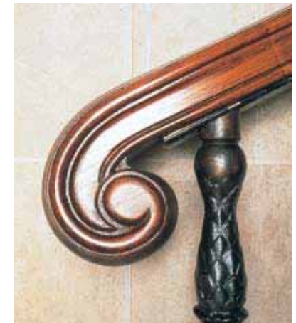
As can be seen with this handrail at the Bank of England, it is possible to form new handrails that match existing designs and materials.
