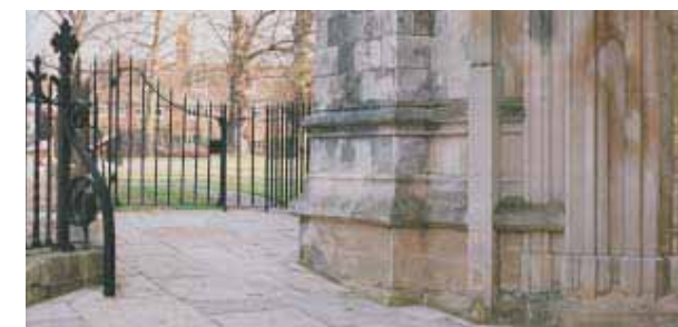
A ramp made from paving stones at the west front of Winchester Cathedral creates an accessible route into the building.
