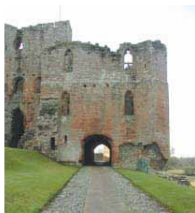
Brougham Castle. Cobbles and setts are particularly difficult for people with limited mobility, especially if they are rough, uneven or open-jointed. It may be possible to create a new route with the use of sympathetic paving stones set within the cobbled or setted areas.
