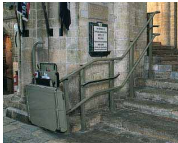
Stairlifts are intrinsically visually intrusive. However, at Winchester Cathedral a stairlift has been carefully positioned at the side of the north transept. The huge scale and complexity of the background architecture help reduce the contrast and visual impact.
