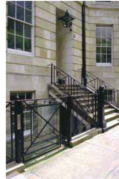
King's Bench Walk, Inner Temple, London. A short-rise platform lift is positioned behind railings where it descends to basement level and connects to the primary circulation routes.
