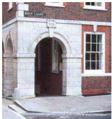
The use of natural stone is retained in the formation of the dropped kerbs in this sensitive location. There is no tactile surface.
