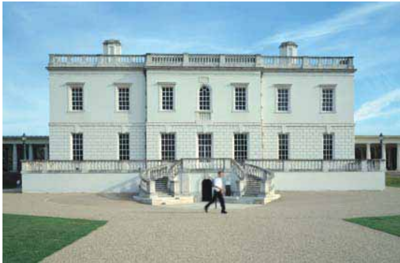
An accessible visitors' entrance has been formed by lowering external levels at the Queen's House, Greenwich. This has involved adding a base to the existing external horseshoe stairs.
