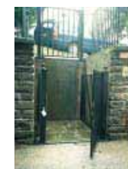
The improved reliability of external lift systems makes them dependable. At St George's, Brandon Hill, in Bristol two external hydraulic lifts provide access at two level changes between the upper churchyard car park and the floor of the church (now a concert hall). The lifts have also proved useful in moving heavier equipment and large instruments.
