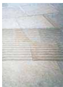
These two photographs illustrate tactile paving formed in natural stone.
