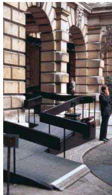
At the Royal Academy the permanent scheme which replaced unsightly temporary ramps involved the modification of the plinth to accommodate the raised courtyard levels.
