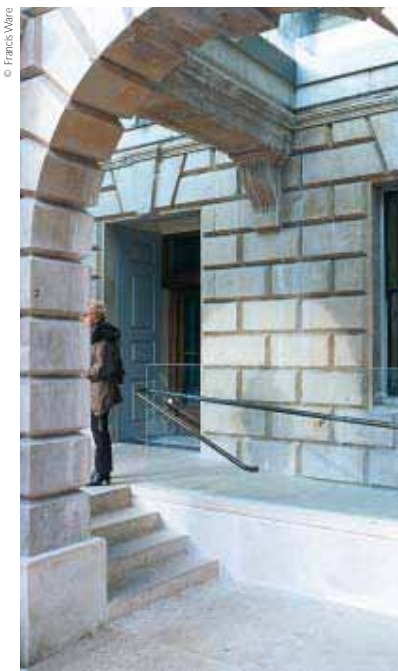
At the Royal Academy the permanent scheme which replaced unsightly temporary ramps involved the modification of the plinth to accommodate the raised courtyard levels.
