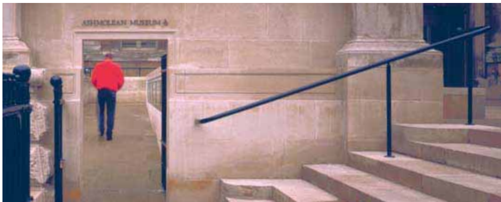
The stone-paved entrance forecourt at the Ashmolean Museum in Oxford incorporates symmetrical access ramps. Particular care was given to the selection and detailing of the stone used in the scheme.
