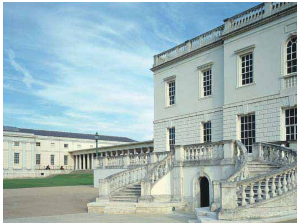
At the Queen's House in Greenwich level access has been provided at basement level by forming a gently dished semicircular forecourt in front of an existing central door opening on the north front. The new paved route forms the access for all public visitors and is not a separate route for people with disabilities.
