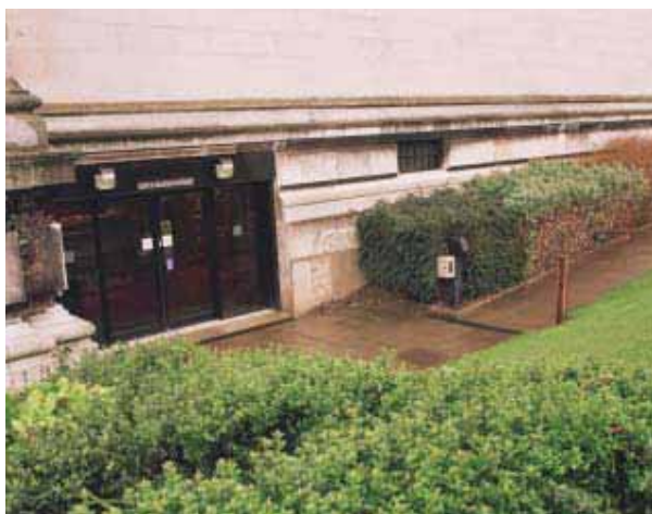
At the Lady Lever Art Gallery in Port Sunlight a new public entrance with a ramped approach has been formed at basement level for all visitors. Adapting the steps to the main portico entrance was considered to be unfeasible.
