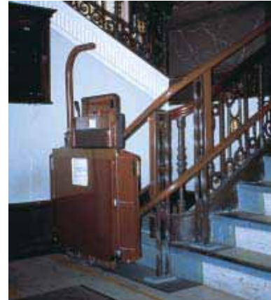
This view of Halifax Town Hall shows how a fine 19th-century staircase can be negatively affected by visual intrusion. As technology develops, more sympathetic intervention may become possible.
