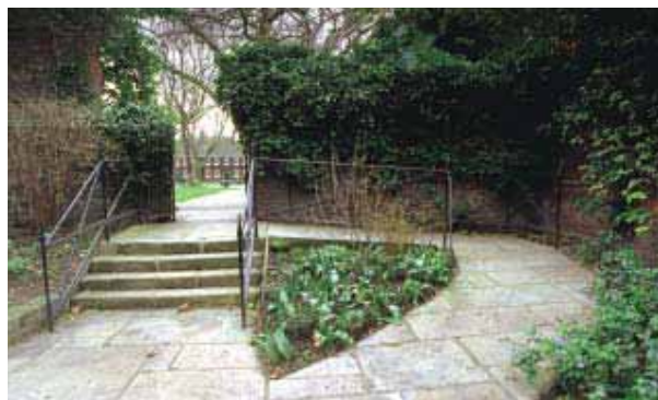
The ramped access at the Geffrye Museum has been designed as part of the sunken herb garden.
