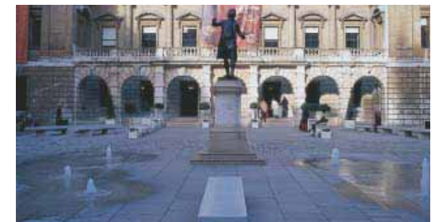
As part of an extensive scheme including full access improvements, the entire courtyard at the Royal Academy has been relaid to a slope to take out the kerb and four steps leading up to the portico. Symmetrical ramps have been inconspicuously inserted along the back wall of the portico to complete the route up to the main entrance.
