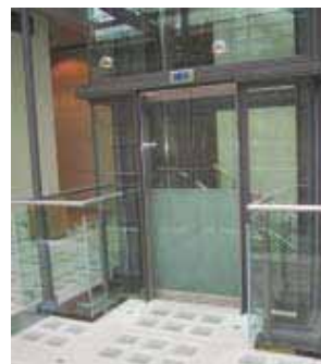
The new 'link' formed in the well between the buildings at the Manchester Art Gallery now contains primary access to buildings. The design of the new passenger lifts and the bridge uses glass in a way that provides good contrast and avoids unwanted transparency.
