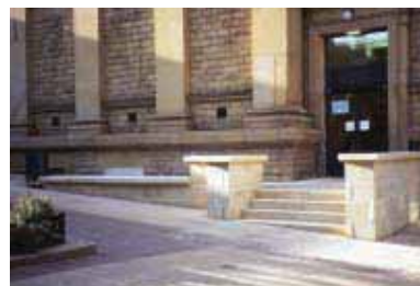
At Morley Town Hall a new level principal entrance has been created at the side of the building to avoid existing stepped entrances.
