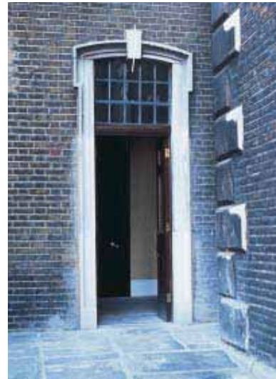
The Christopher Wren-designed church of St James sits between Piccadilly and Jermyn Streets, which are at different levels. Level access has been achieved from Jermyn Street by altering a window to form a doorway, which is located in a 19th-century addition to the original body of the church and deemed less sensitive. It was not possible to make adjustments for the level change from Piccadilly.
