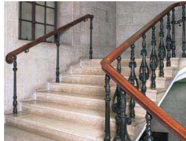
As can be seen with this handrail at the Bank of England, it is possible to form new handrails that match existing designs and materials.
