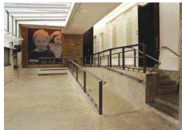
New access improvements at the Almeida Theatre have been incorporated as part of a larger project. A new foyer ramp provides a non-stepped approach to the stalls seating area.
