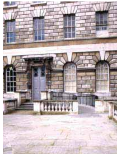
The stone balustrade has been cut through on one side of the entrance to the Seaman's Hall at Somerset House to provide a ramped access.
